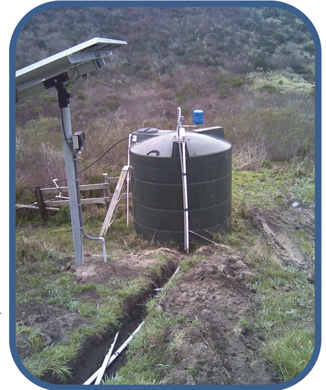
Stock Watering System with a solar powered pump to fill a small tank which then gravity feeds to a trough. Photo credit John Warner.
